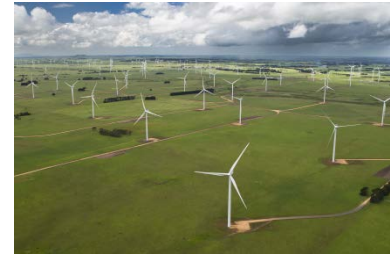
Site infrastructure / Balance of Plant
