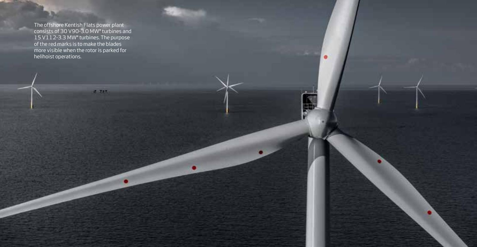
The offshore Kentish Flats power plant consists of 30 V90-3.0 MW\* turbines and 15 V112-3.3 MW\* turbines. The purpose of the red marks is to make the blades more visible when the rotor is parked for helihoist operations.
