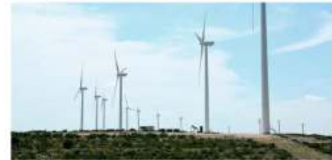
Vestas secures its largest service contract renewal for 1,897 MW
