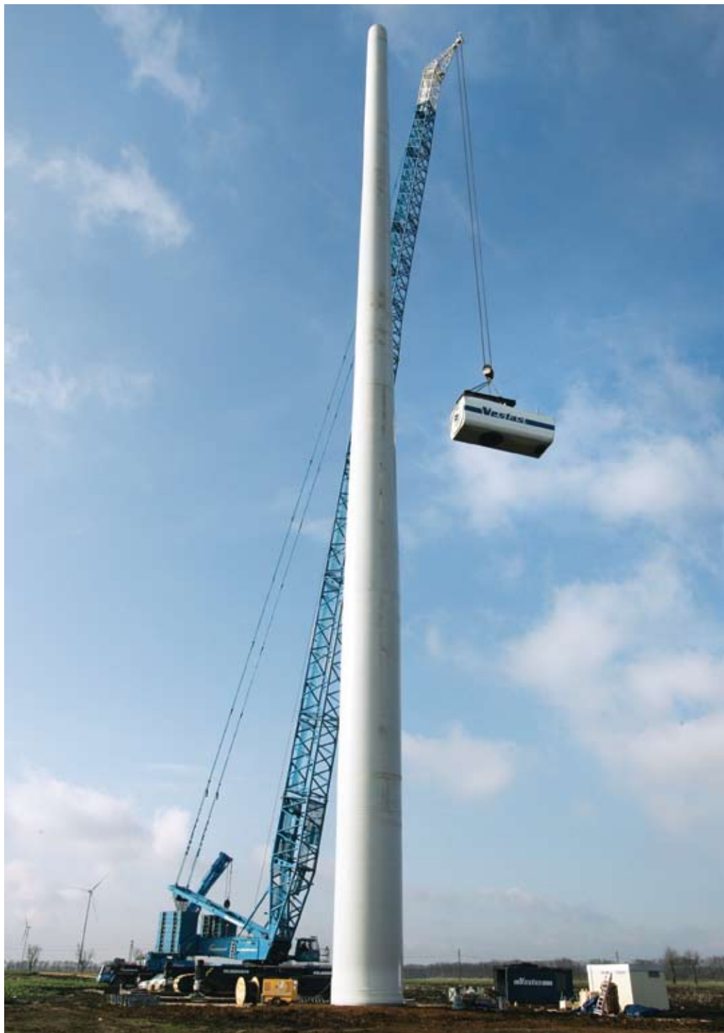
Construction of wind farm in Kavarna, Bulgaria ▶
