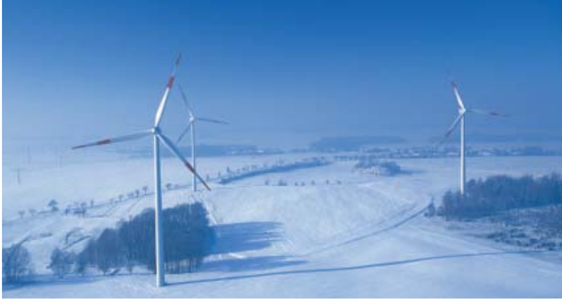
The Puschwitz wind farm in Germany consists of ten V80-2.0 MW turbines.
